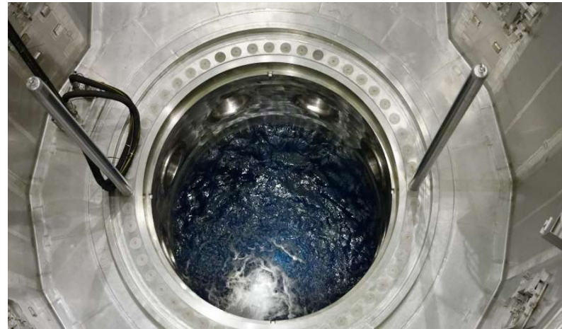
Reactor pressure vessel circuit cleaning
