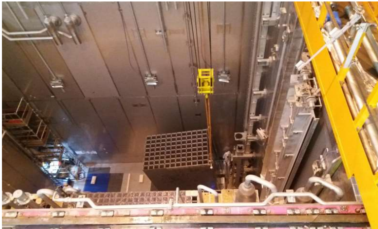
Fuel rack installation within the pool
