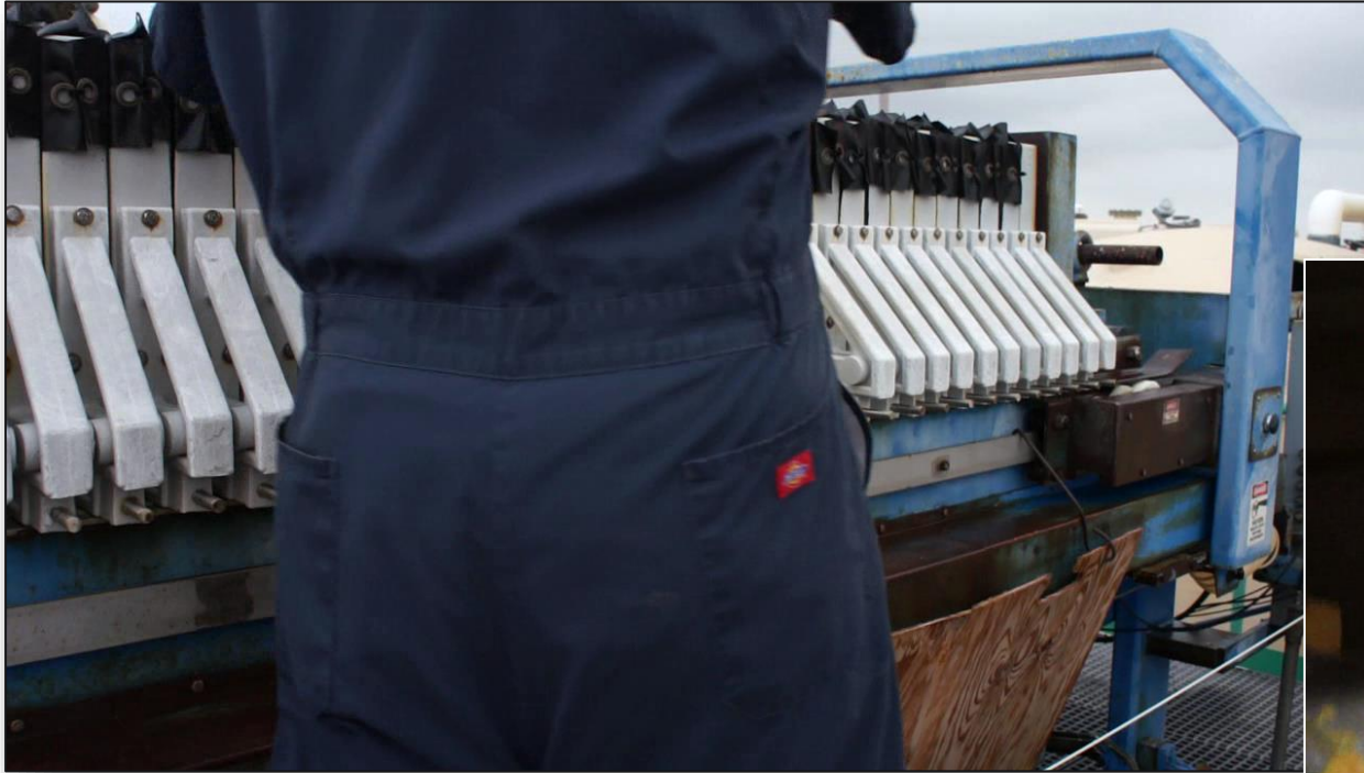
Yellowcake Filter Press, UEC Hobson Processing Plant, Texas
